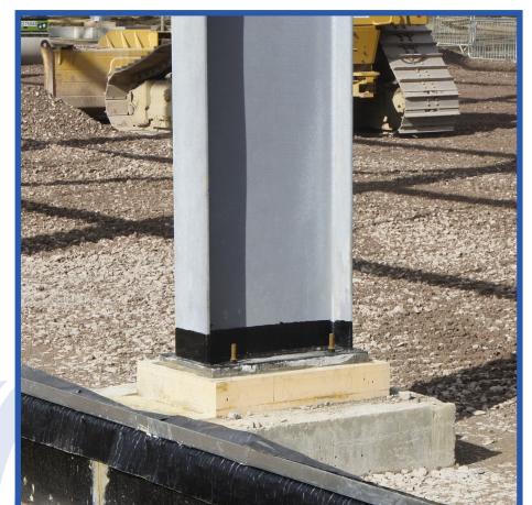
Column Base Thermal Break
