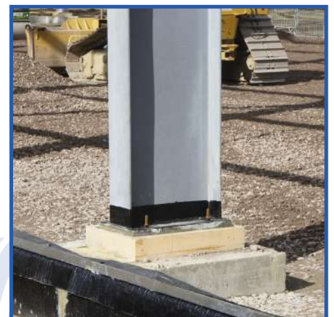
Column Base Thermal Break
