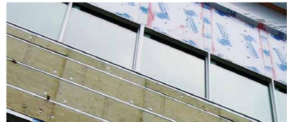
Exterior insulation installed in-between steel z girt cladding support attachment resulting in exterior insulation that is not continuous and does not meet energy codes (Source: Roxul, Inc.)
